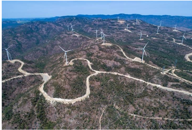
Figure 1: Mount Emerald Wind Farm, Qld, showing the clearance required for pads and tracks.
